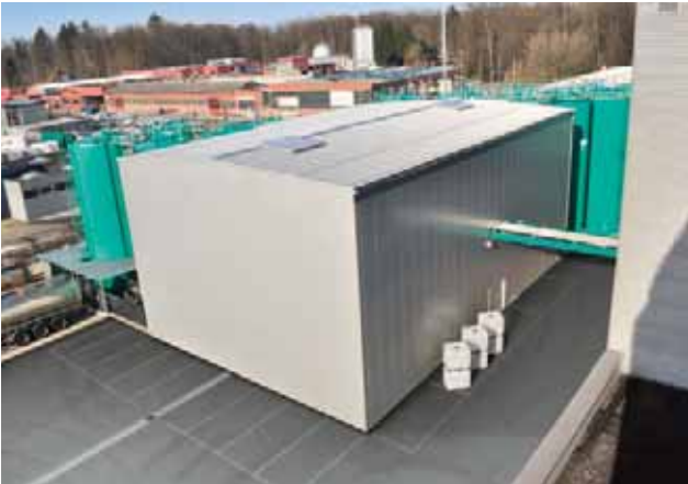
With the new fully enclosed storage tanks with pigging technology, Motorex emphasises once again its dedication to quality as leading Swiss lubrication technology specialist.
